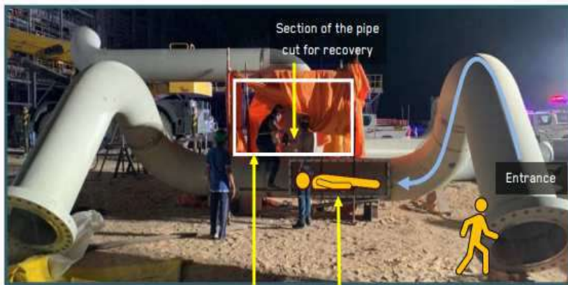
Area where welding was performed
